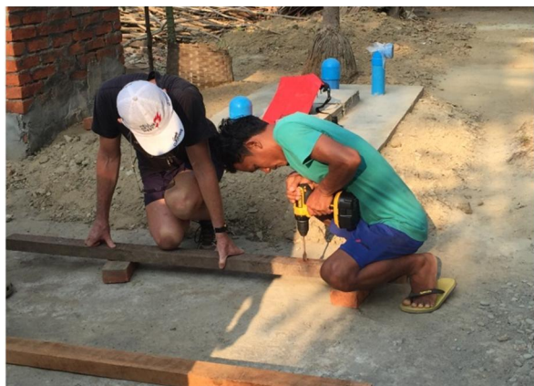
Htein Lin drilling the roof battens with Graeme lending a hand.
