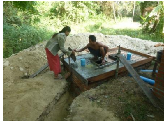
Septic tank lid being poured
