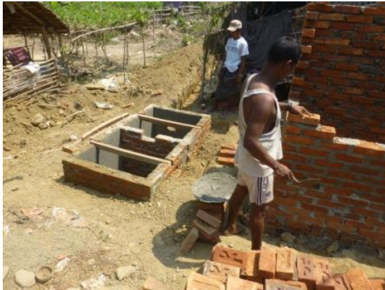
Building a toilet in the village
