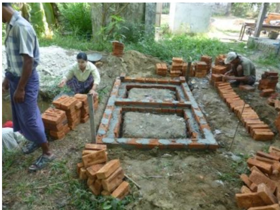
Footings for the school toilet building
