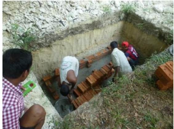
Septic tank hole dug, the work begins
