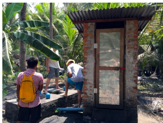
Inspection one of last years toilets
