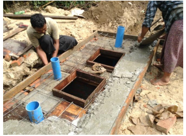
Pouring the septic tank lid.
