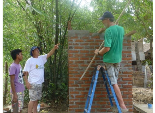
Fixing the roof frame. Greg directing while Thein Lin watches on.
