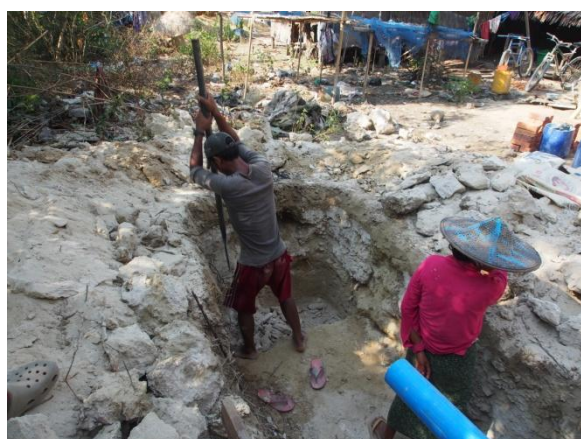
Workers digging the hole for the septic tank. Yes, that's a girl helping!
