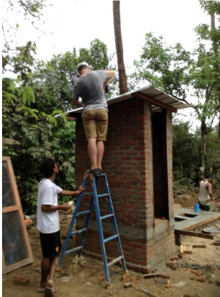
Jamie fitting the roof sheets.
