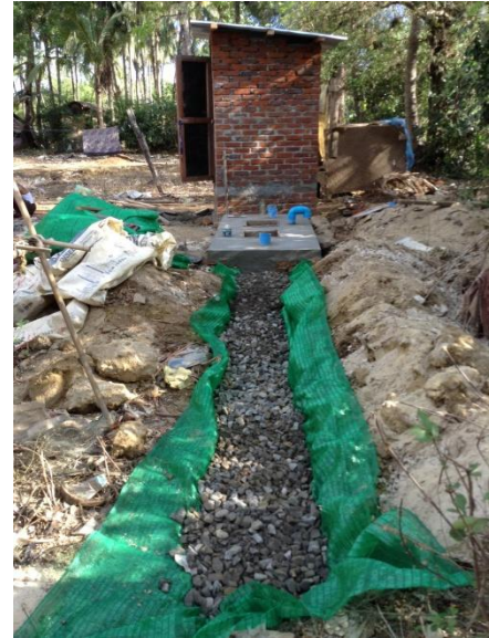
Installing the absorption trench.
