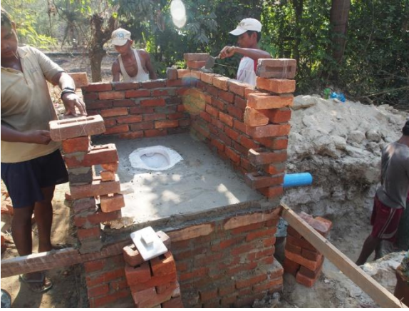
Building the toilet.
