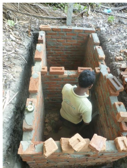
Building the septic tank.
