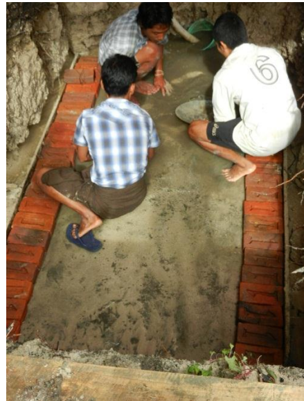
1 st course of wall bricks.
