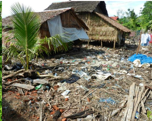
Rubbish dumping under and around housing
