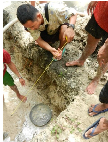
Water constantly enters the hole, emptying soil "a wok at a time". Measuring overall depth.
