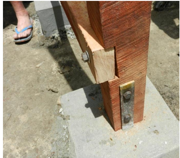
Posts bolted into position.
