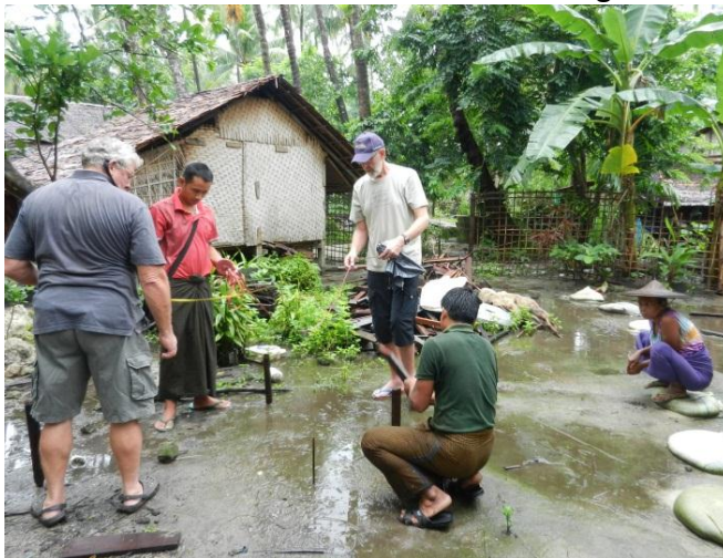
Pegging and measuring the site.
