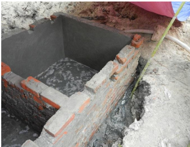
Fully rendered septic tank.
