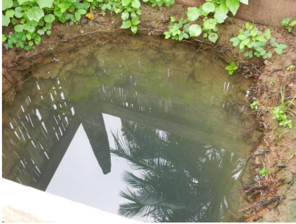
Some wells are not lined and just earthen walls
