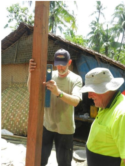
Ensuring the posts were plumb.
