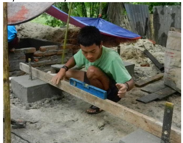
Footing poured and checked.
