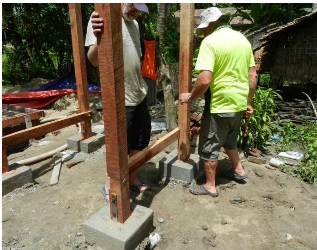
Ensuring the posts were plumb.
