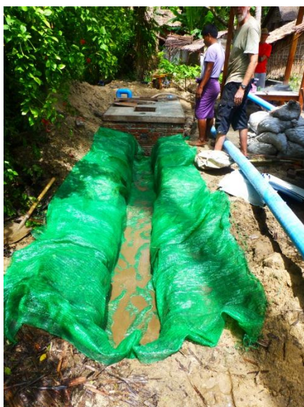
Woven fabric to stop the pipe silting up, slotted pipe bedded in gravel and wrapped in fabric
