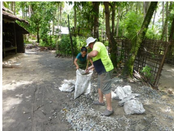
Bagging the gravel to carry to site.
