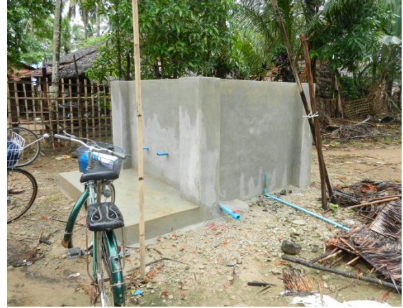
New water tank under construction
