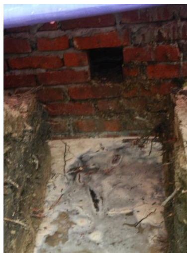
Hole in side of septic for slotted overflow pipe.
