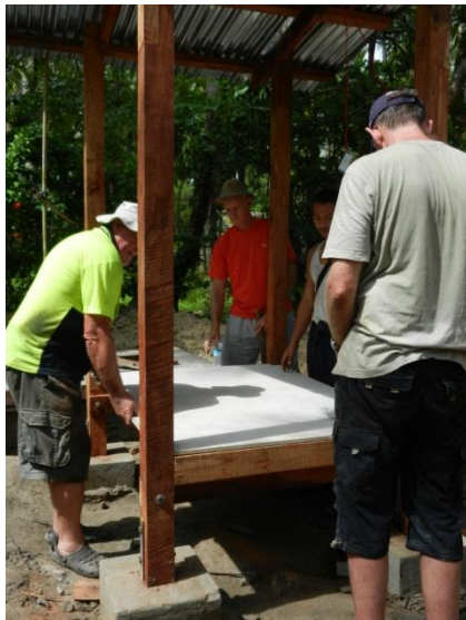
Compressed flooring in position.
