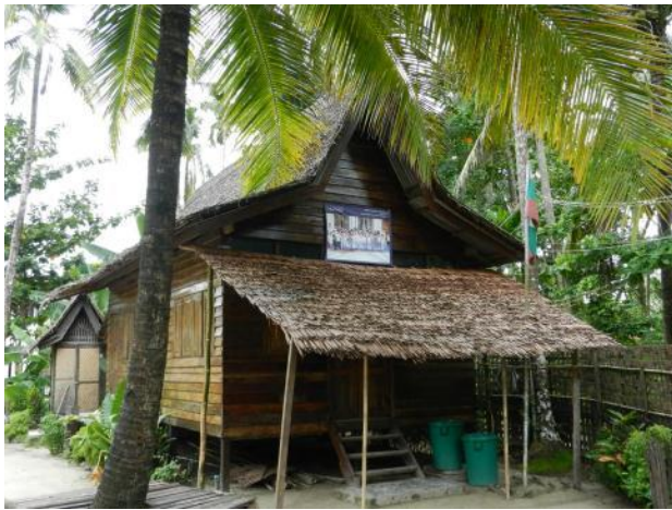
The original school building built by Mamma Sue and the Andrew Clarke Foundation
