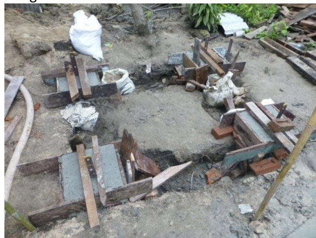
Footings boxed up and poured.
