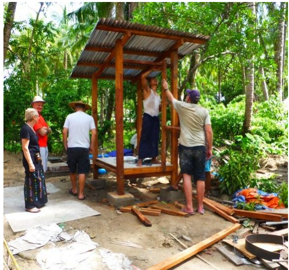
Finishing the timber work.
