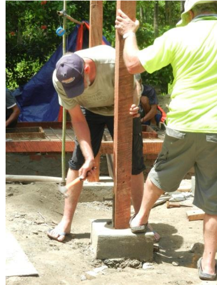
Fixing the timber posts to steel stirrups.
