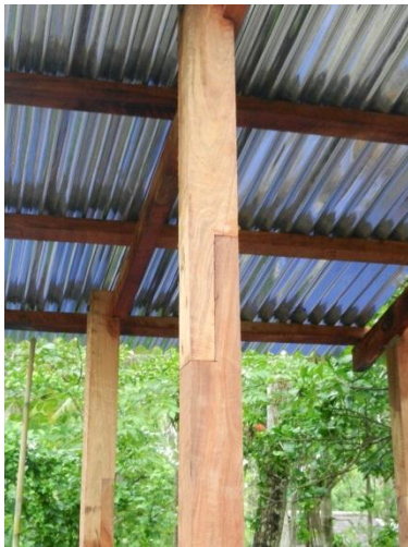
Posts in position and joined and roof affixed.
