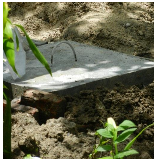
Septic tank hatch cover poured and ready.
