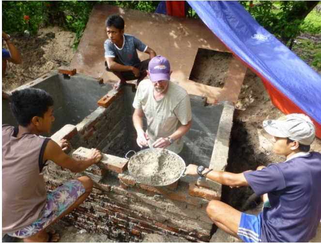
Rendering the inside of the septic tank for water proofing.
