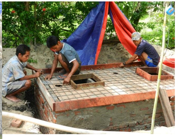
Fixing reo for the concrete lid.
