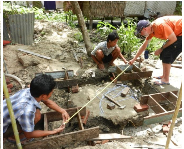
Geoff measures the footings. Note the Myanmar safety boots!!!
