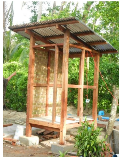
First side wall installed.
