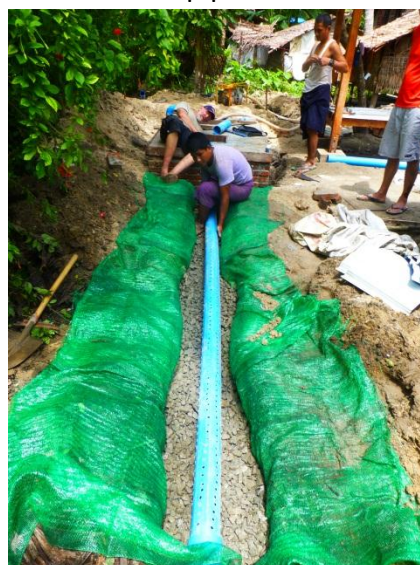
Woven fabric to stop the pipe silting up, slotted pipe bedded in gravel and wrapped in fabric
