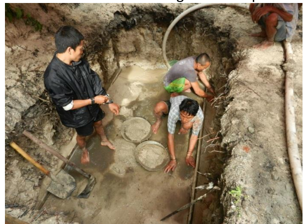
Site covered with tarp to keep out rain. Concrete mixed for base slab. Putting in timber formwork for base slab.
