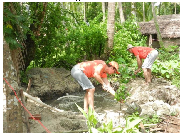
Anne and Terry backfilling the old hole.
