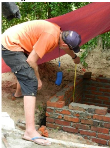
Geoff checking final height of walls.
