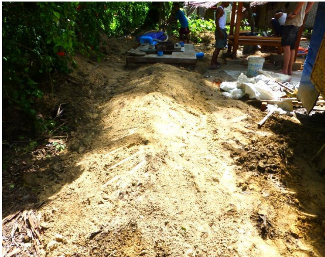
Trench backfilled .
