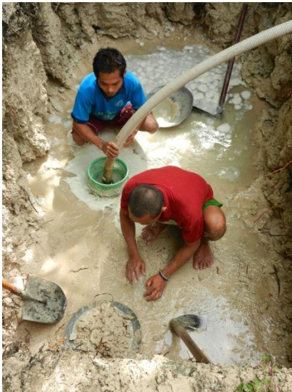
Water constantly enters the hole, emptying soil "a wok at a time". Measuring overall depth.
