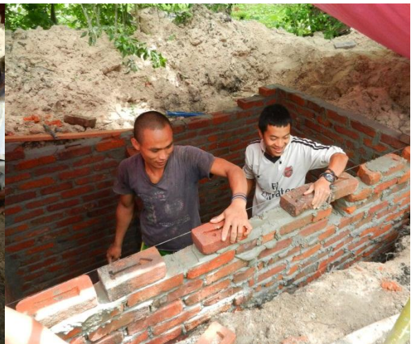
Tank taking shape.
