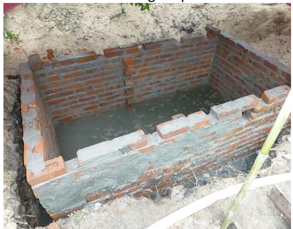
Work on dividing wall commences.
