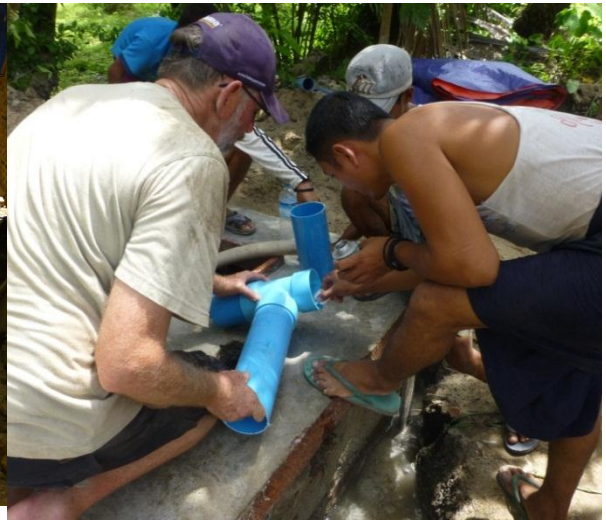
Gluing plumbing pipes for installation.
