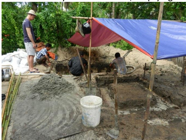
Site covered with tarp to keep out rain. Concrete mixed for base slab. Putting in timber formwork for base slab.
