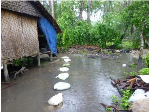
The site underwater and with sandbags to stop us getting bogged in the mud with our thongs.
